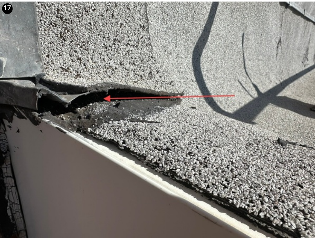
Failed flashing seam and large open condition--typical.
